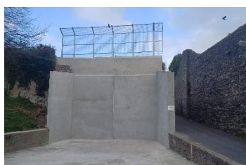
Handball Alley refurbishment
