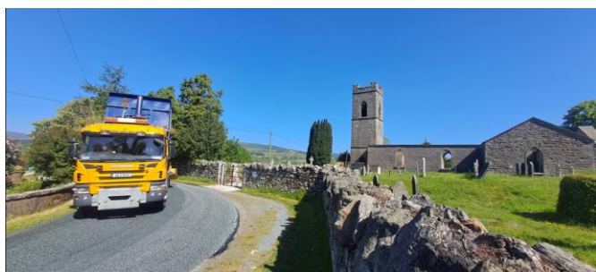
Surface dressing at Derrylossary, Roundwood.
