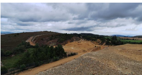
New perimeter fencing at Avoca Mines East
