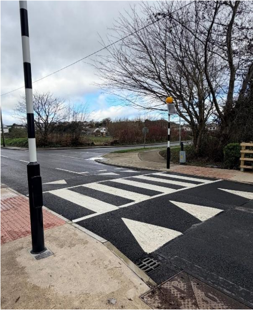
Before and after photos of the Kenmare Heights footpath renewal scheme at location prone to flooding
